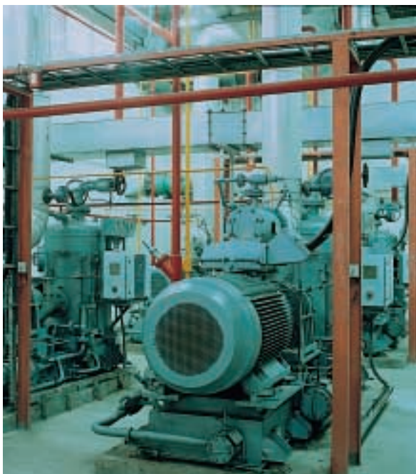
Complete ammonia refrigeration plant installed at an ice cream factory in China. Screw compressors, made by Grasso, are the heart of the installation.
