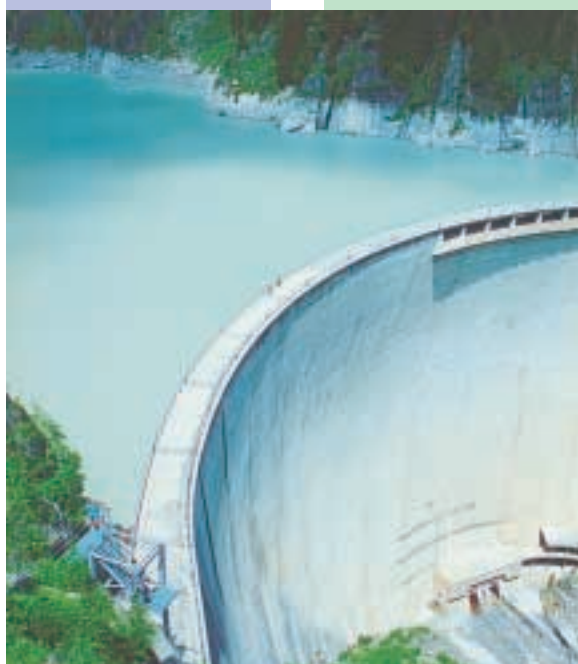
The addition of chilled water or ice to a concrete mixture provides a better control over the hardening process of dams.
